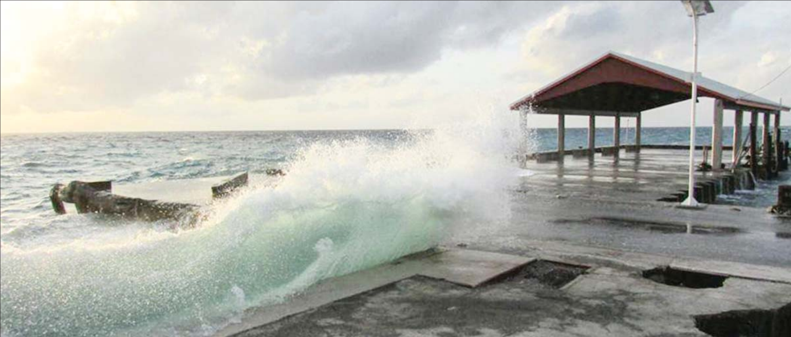
West winds throw waves against the Ebeye Pier early last week.
